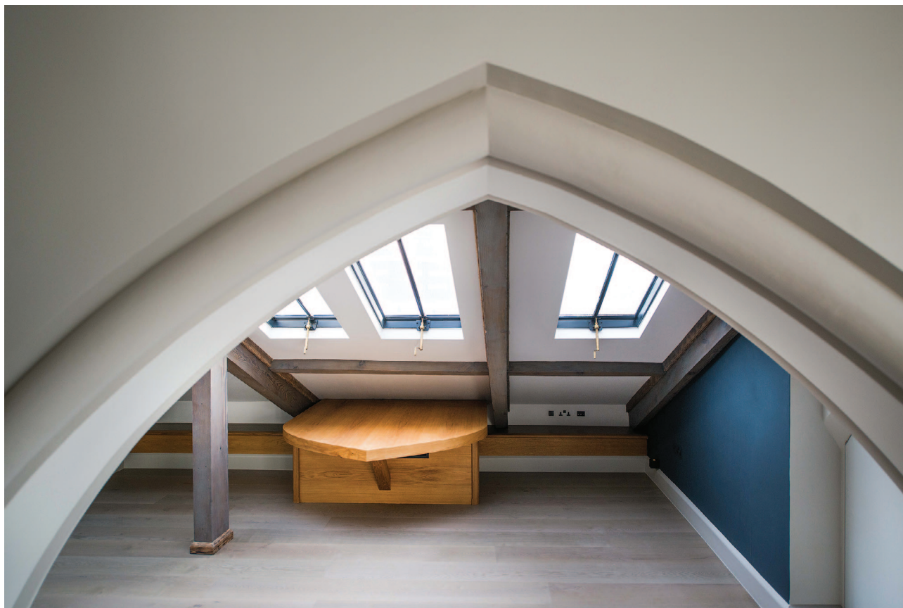
Above, Various Clement rooflight sizes were chosen for The Sanctuary in Battersea. Clement 6 rooflights are shown here - their long rectangular shape creates a major design feature.
