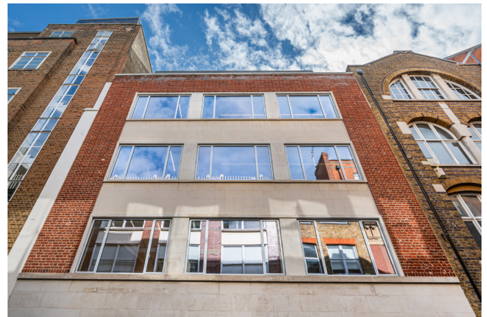
Above, the Jansen windows and doors by Clement at Little Portland Street improve thermal and air tightness at the building.
