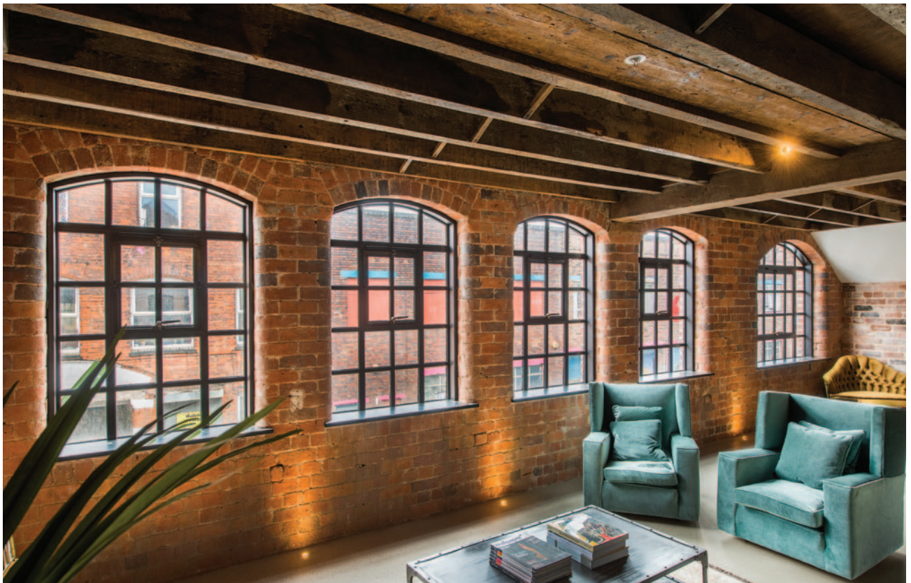
Above, new double glazed steel windows by Clement at Comet Works, Birmingham
