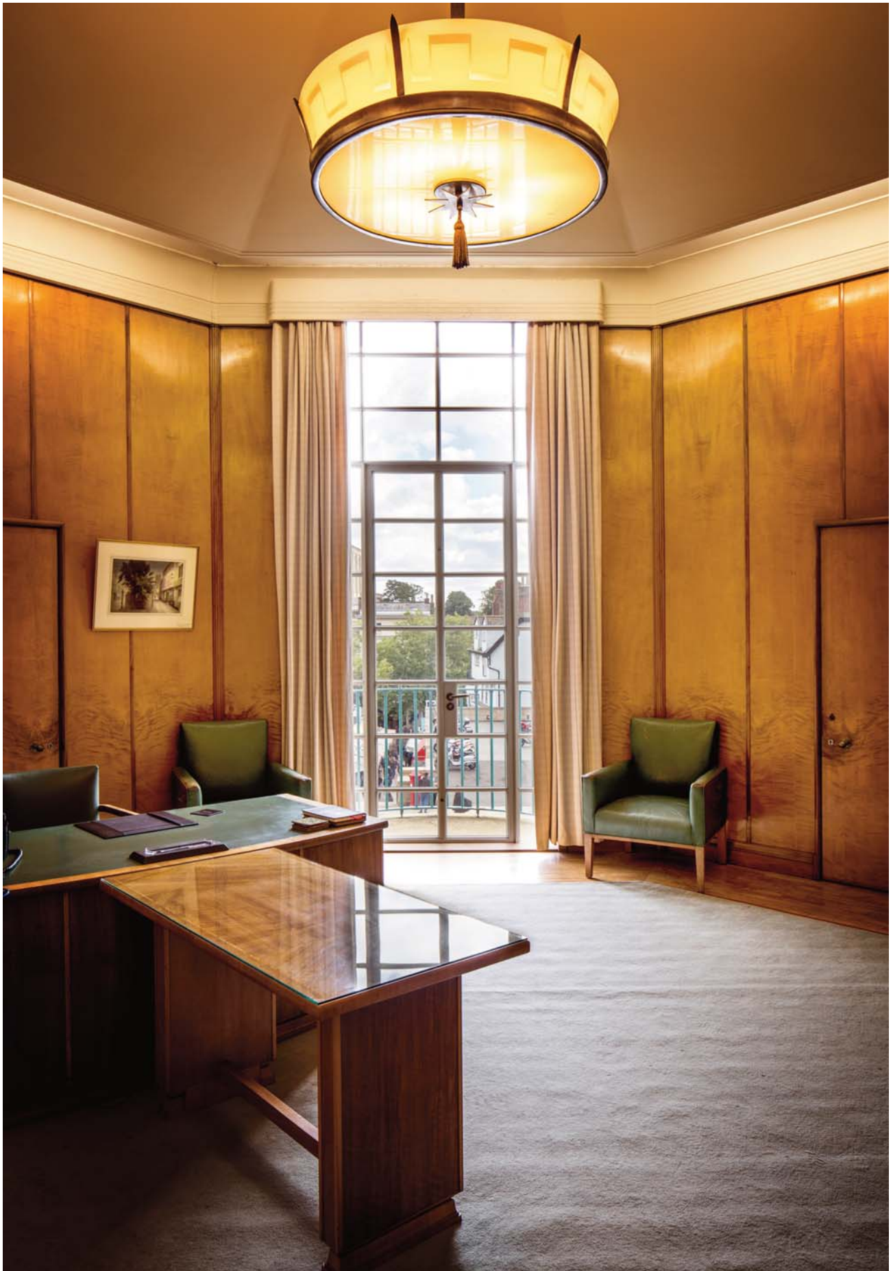
Above, the new steel windows mean improved energy efficiency and security for Norwich City Hall whilst still retaining the original character of the building.
