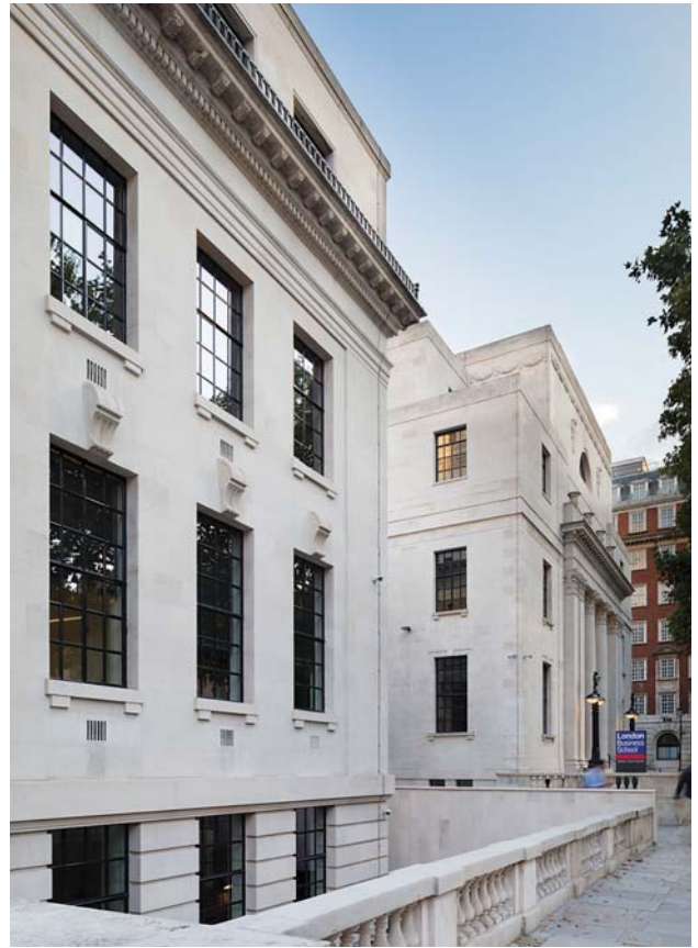
Above, New steel windows from the Clement EB24 range at Old Marylebone Town Hall featuring specialist glazing for better acoustic and solar control
