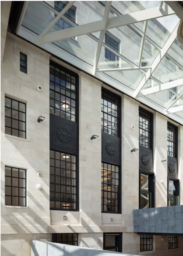
Above, New steel windows from the Clement EB24 range at Old Marylebone Town Hall featuring specialist glazing for better acoustic and solar control
