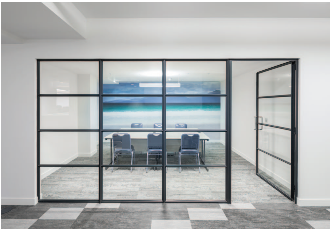
Above, Clement W20 suite of steel sections with genuine T bars in RAL 7016 (Anthracite Grey) at 188 Fleet Street in London
