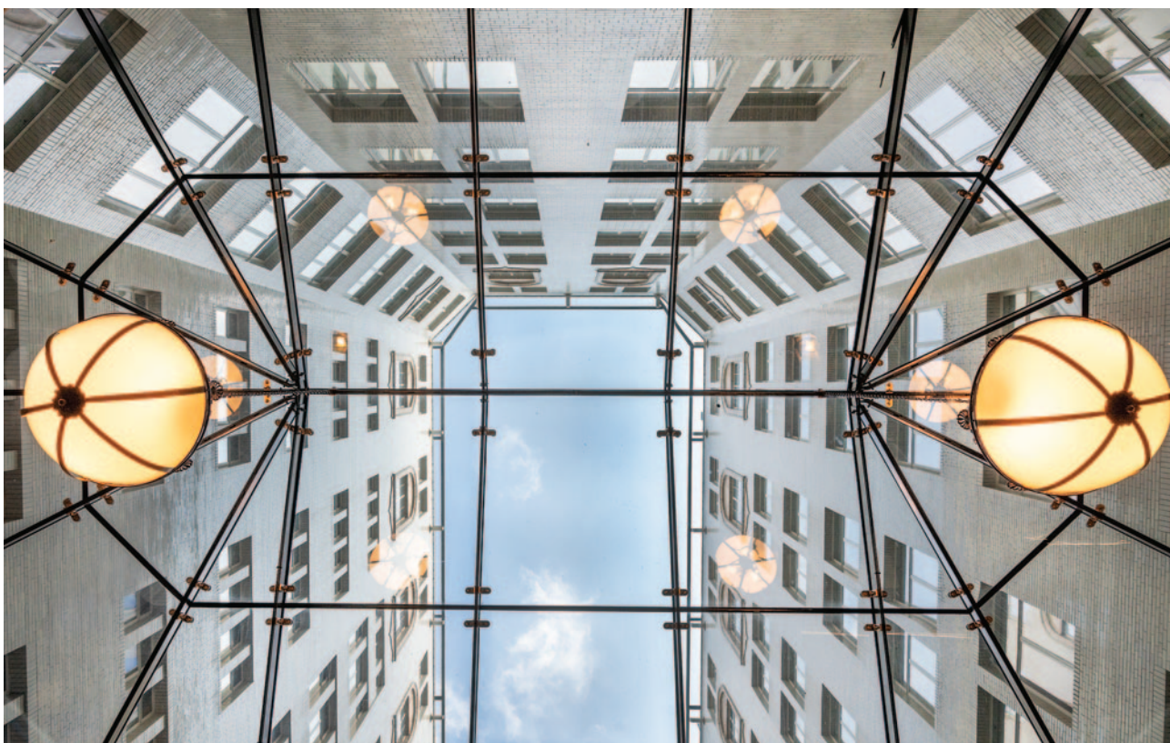
Below, the new steel windows at the India Buildings provide a close match to the originals while offering improved thermal performance
