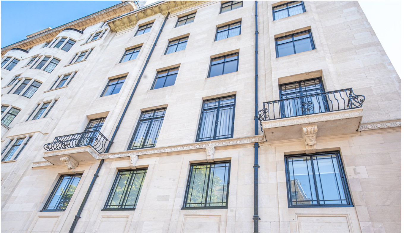
Above, New Clement EB24 steel windows provide the perfect match to the Art Deco fenestration at this Georgian-fronted apartment building in London
