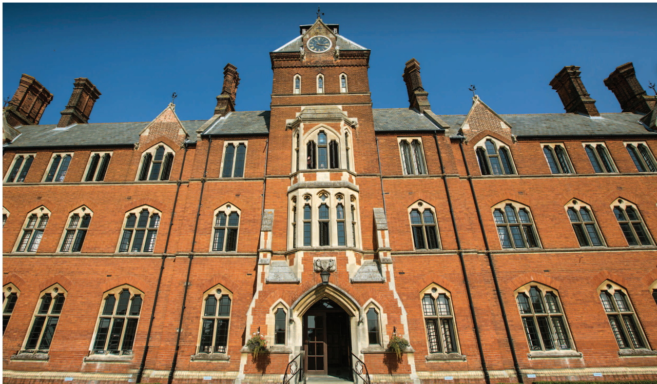
Above, Clement W40 steel windows at Framlingham College
