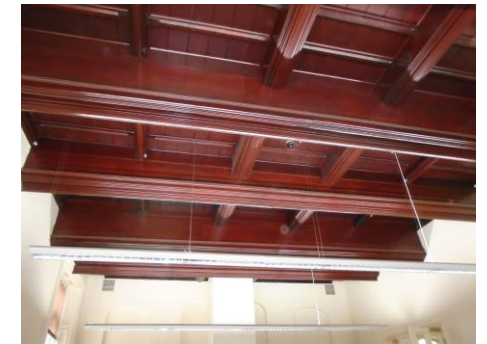
Underside 1 st Floor Court
