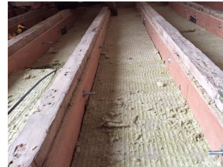
Structural Ply Joist Strengthening
