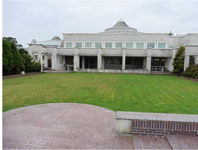
East Elevation from landscaped gardens
